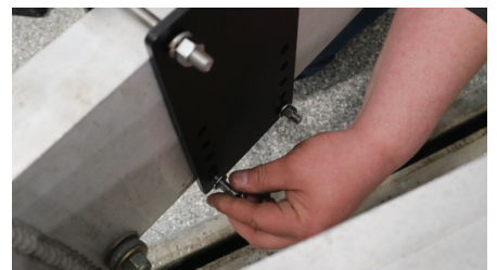
Figure 4: Find desired height and insert the remaining long carriage bolts, washers, & nuts.
