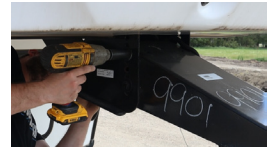
Figure 1: Losen pin box bolts & nuts and remove original pin box
